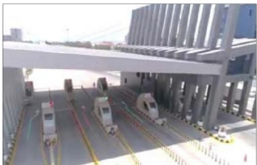
■ The new electronic payment system at the causeway
